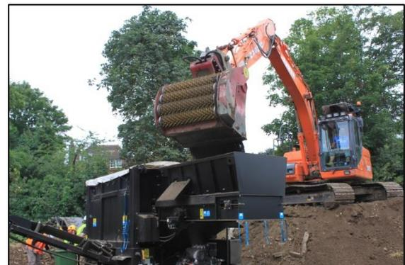
*Photo 2 - Loading the Xtract machine for on-site processing of knotweed infested soils*
